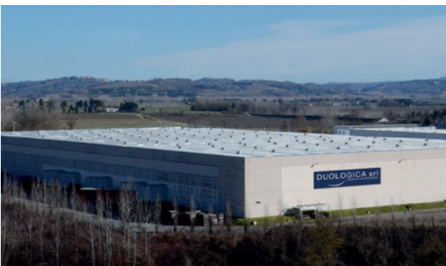
Full Wi-Fi Coverage in the Warehouse of Duologica Srl, an Italian Logistics and Distribution Company
