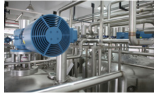
Industrial Automation Control Systems
