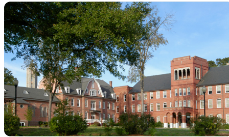
Outdoor Wi-Fi Backhaul for Large Campus
